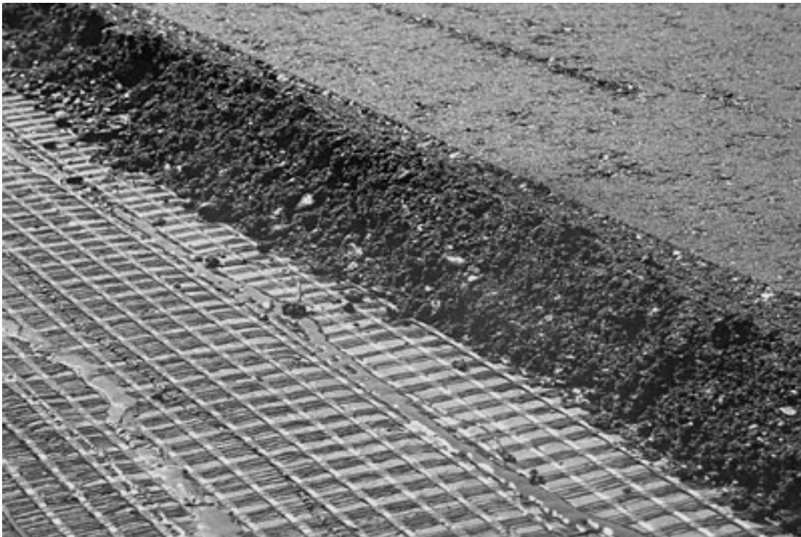
Figure 5. The construction of reinforcing asphalt pavements
